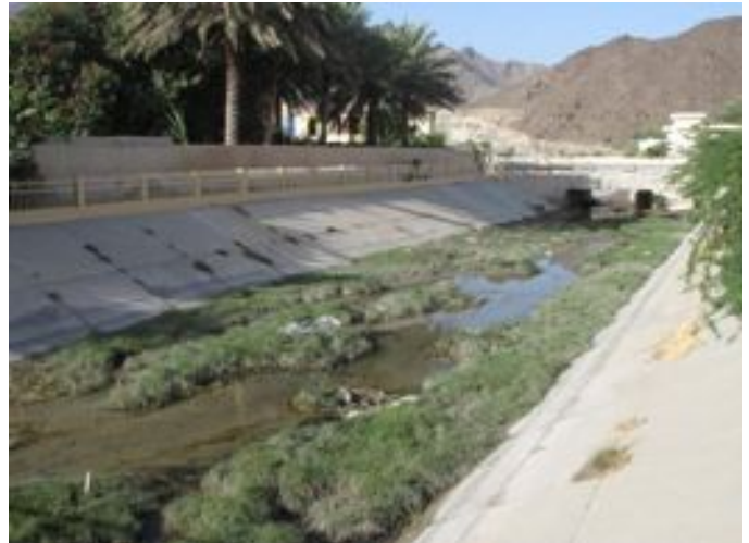
The situation in the middle reaches of the channel has created islands with vegetation
